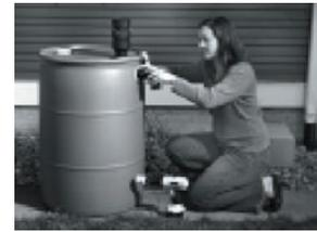
**3 Foundation:** Create a raised, stable, level base (like concrete blocks) for the rain barrel to sit on. You might want to test stability by filling the rain barrel with water before attaching to your structure. A full rain barrel is very heavy and tipping is a risk if it's unsecured or on an uneven surface.
