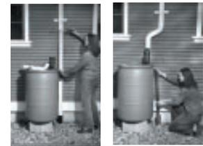
**Attach Barrel:** Set up the barrel beneath the elbow and secure the barrel to the house with a strap. Cut and attach the overflow pipe to the overflow elbow and direct to the existing discharge location.
