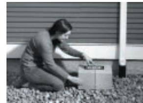
**4 Downspout:** Cut the downspout with a hacksaw so that the elbow will sit just above the rain barrel inlet. Attach the elbow over the downspout with a screw and secure the downspout to the house with the strap.
