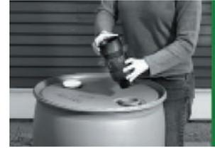
**2 Overflow:** Drill a hole near the top of the barrel to accommodate an overflow pipe that is at least 2 inches in diameter. If the overflow pipe elbow seals and seats securely, it can be threaded directly into the barrel opening. If not, it should be secured with washers on both sides of the barrel and a nut on the inside. Use Teflon tape around the threads and a bead of silicon caulking around the opening to ensure a tight seal.
